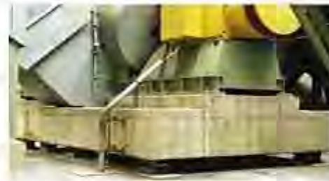
Fig. 6.3.3a—Isolator-supported fan foundation (photo courtesy of GERB Vibration Control Systems, Inc.)
